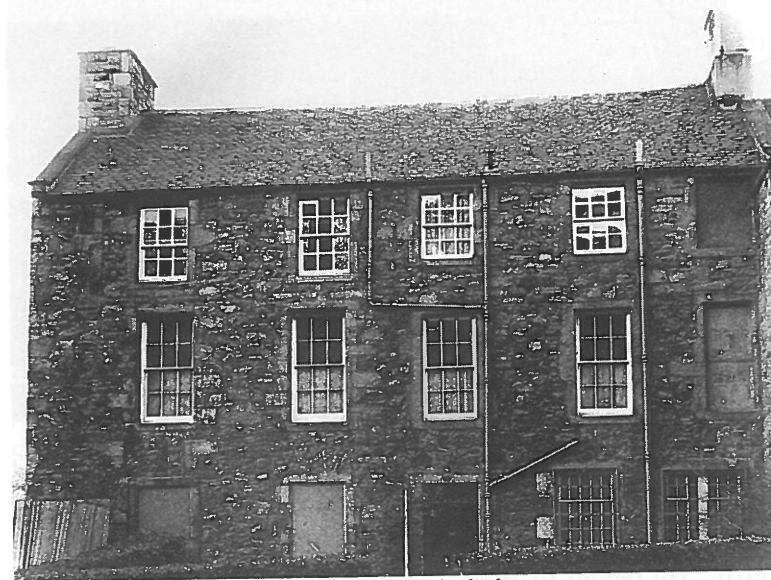
21 St John Street, Edinburgh, before conversion
