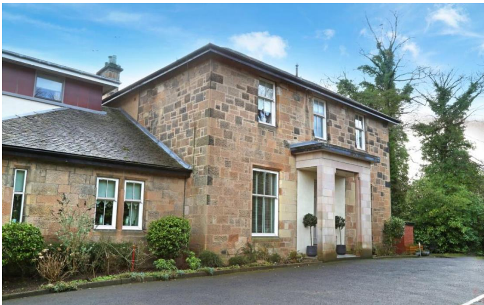
St John Residential Home, Langside
